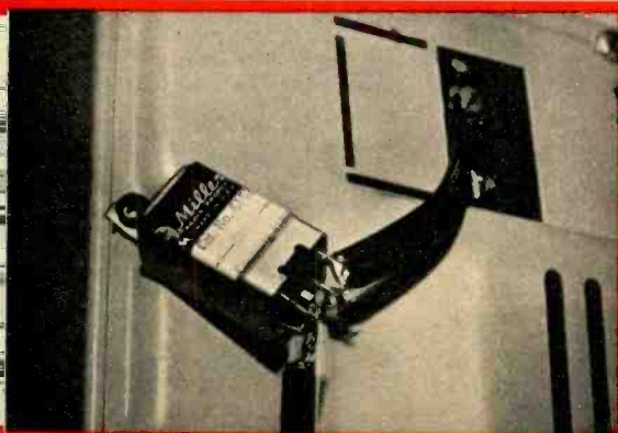
Other transformer is fastened to rear of TV set. Short length of twinlead goes from set's terminals to 300-ohm lugs on the transformer.
