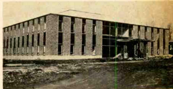
New ARRL headquarters building will be completed about the time this issue of EI appears.
