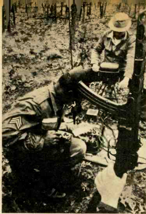
U. S. Special Forces team using a hand-operated generator to power a knee-key CW transmitter.
