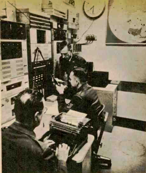
Single-sideband communications room in the SAC cave controls world-wide SSB net. Pins on the polar map on back wall indicate stations in net.
