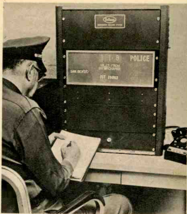
Receiver interprets coded signal, flashes information in lighted letters on panel. The system can be used for telemetering purposes.
