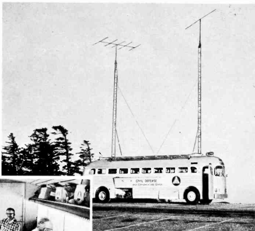
A self-contained net control station on wheels is operated by the Winston-Salem (N.C.) Amateur Radio Club in cooperation with the county's Civil Defense organization. Beam antennas are easily collapsed.
