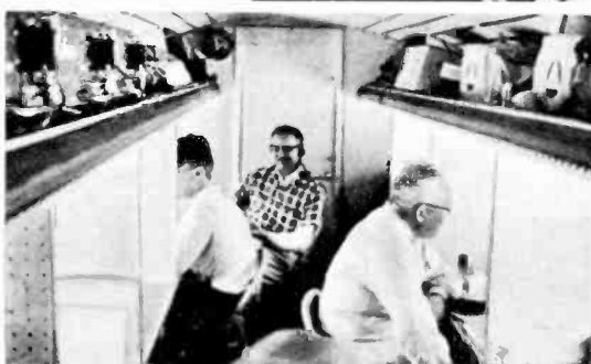
A self-contained net control station on wheels is operated by the Winston-Salem (N.C.) Amateur Radio Club in cooperation with the county's Civil Defense organization. Beam antennas are easily collapsed.
