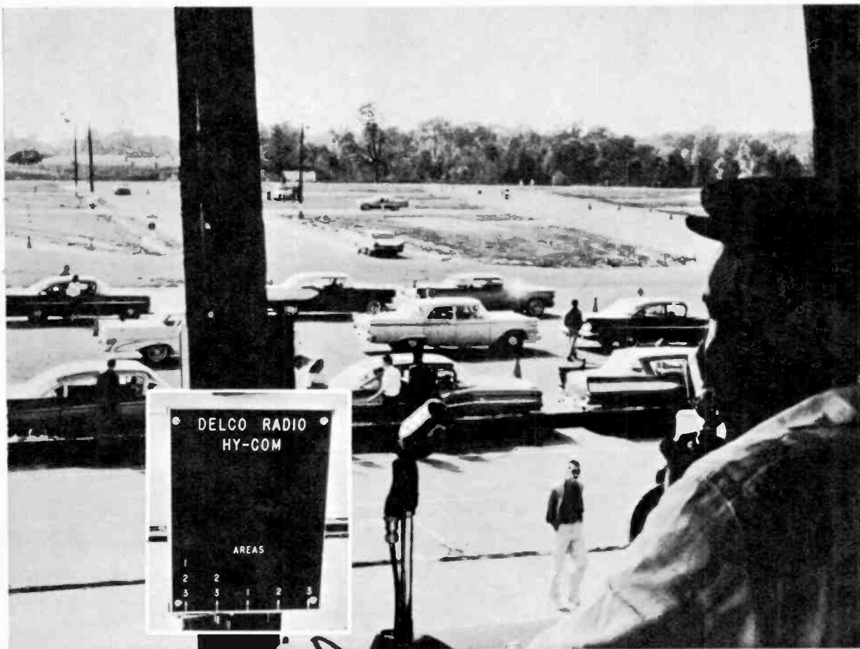
Instructor in tower has a clear view of the entire range. The small Hy-Com panel allows him to talk to one, two or all three areas of the course at once.
