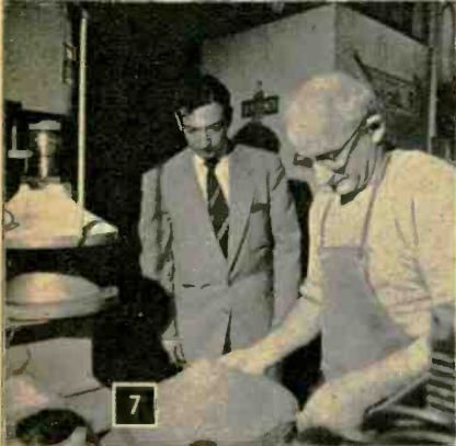
7. Dried cone is peeled off form. Paper at apex is thicker than at rim.
