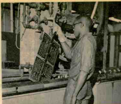
Series of baths remove foreign material that may be clinging to boards, deters corrosion.
