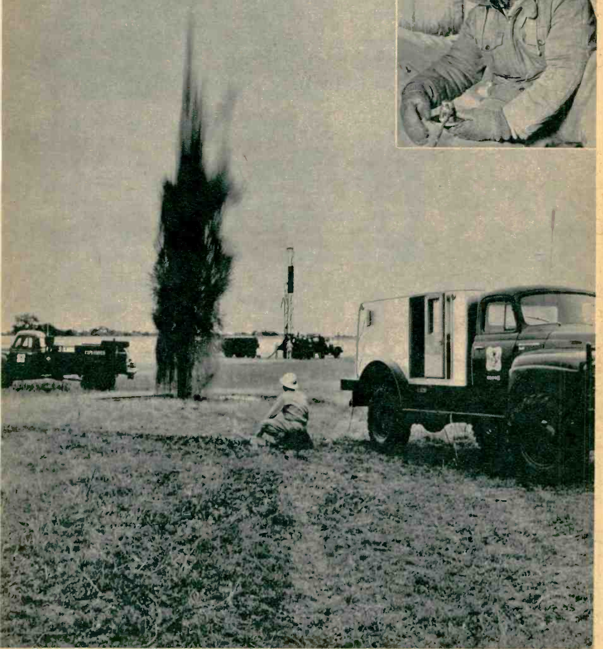
Boom! Dynamite, buried some 45' deep, is exploded to create seismic waves which will penetrate through many strata to bedrock. Rig in background drills holes for insertion of dynamite.
