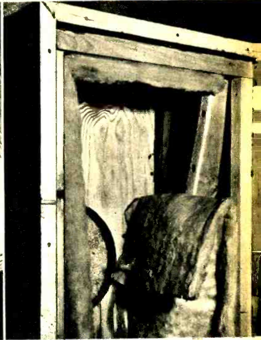
Interior view shows diagonal strip to prevent vibration, and fibreglass damping material.
