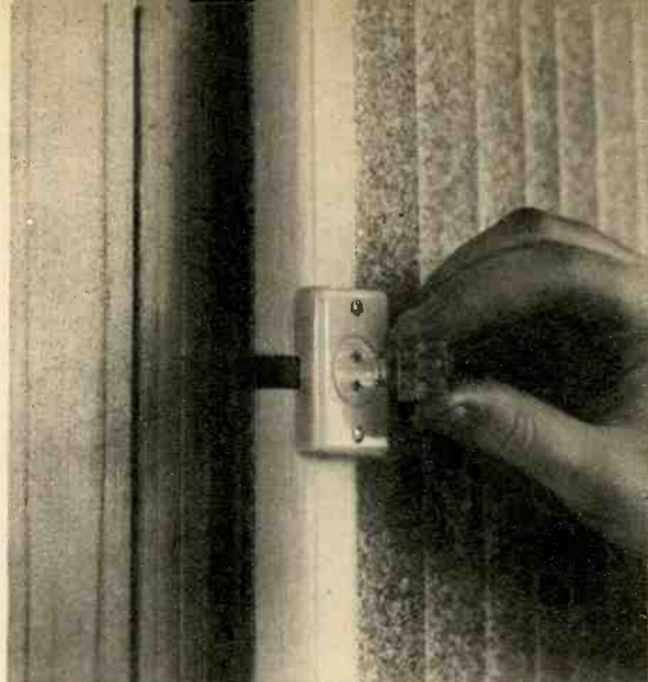
The TV type twinlead plug and receptacle may be mounted at convenient spot outside house.
