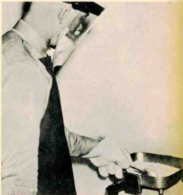
Col. Parkin, wearing protective clothes, stirs cooking fuel with a non-sparking metal spoon.
