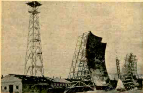
Huge "movie screen" antennas of "White Alice" send radar signals over the horizon.
