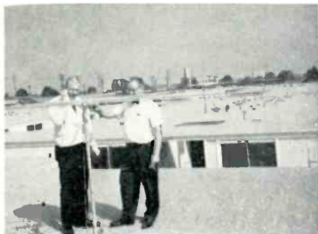
Bill Wesenberg, of Kiesub Corp., left, and George Irwin of Signal TV, in Long Beach, are shown here outside the Park Avenue Apartments. Signal TV installed a master antenna system in these units by using 55 Channel Master 3604 antennas and 4-set couplers to supply 220 individual apartments.
