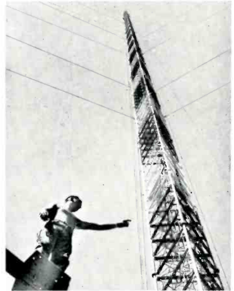
Engineer Al Kivisto motions to the hoist operator.
