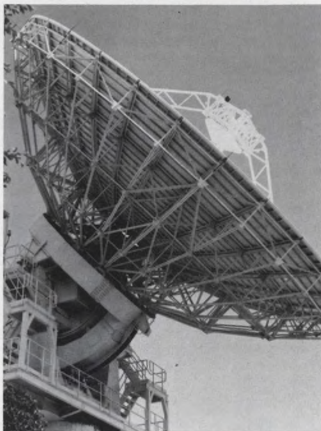
Satellite communications antenna is located at Philco-Ford Corp.'s WDL Div. in Palo Alto, CA.
