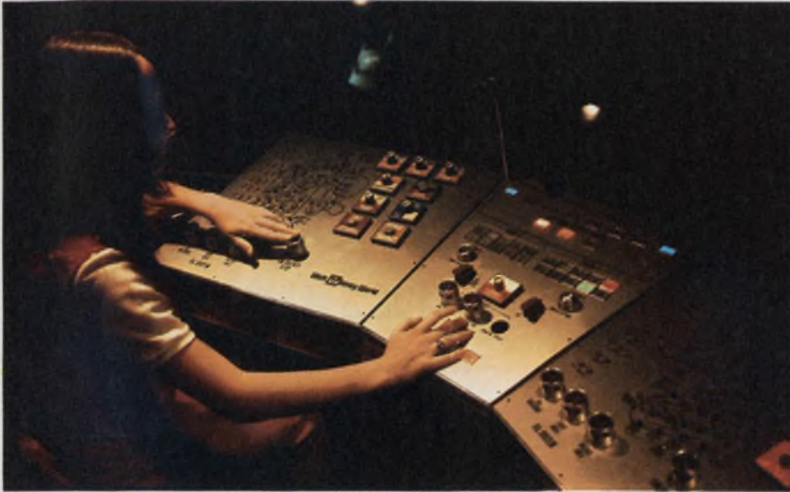
The control room for the Space Mountain thrill ride keeps tabs on the position of every car through magnets along the track and a Nova 2 computer. If cars begin to tailgate dangerously, the whole ride can be shut down.
