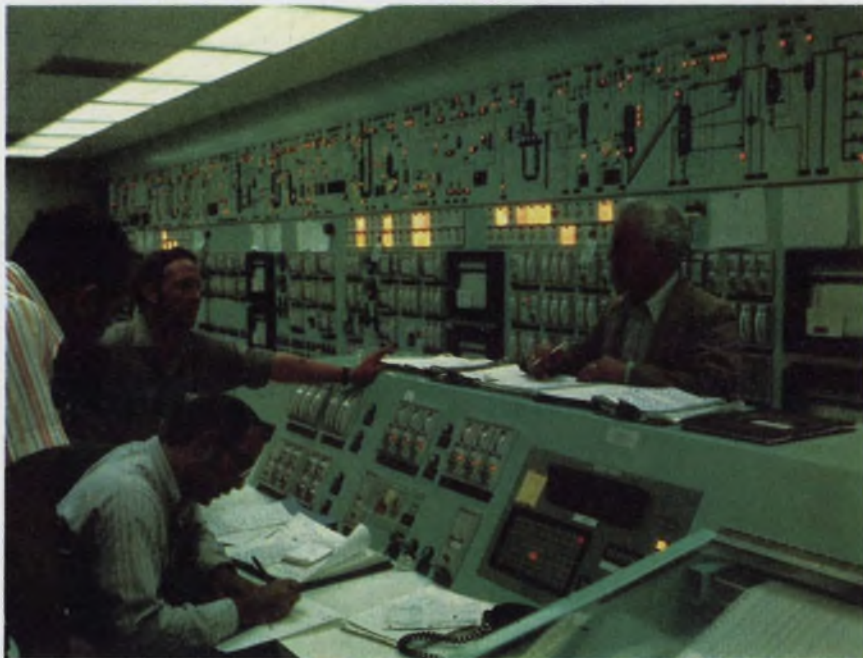
The delicate process of revitalizing used nuclear fuel is displayed in this control room in General Electric's Midwest Fuel Recovery Plant, Morris, Ill. A GE 4020 process computer logs the operation but does not control it.
