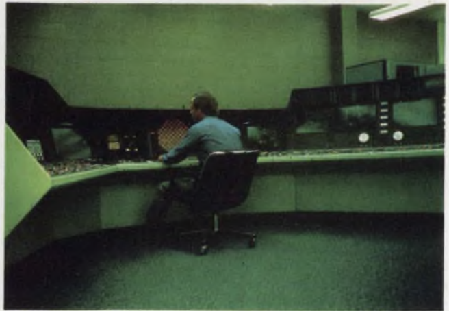
For the future, GE's Nuclenet 1000 control complex uses computer-driven CRTs to replace the hundreds of display meters that now line long control-room walls.
