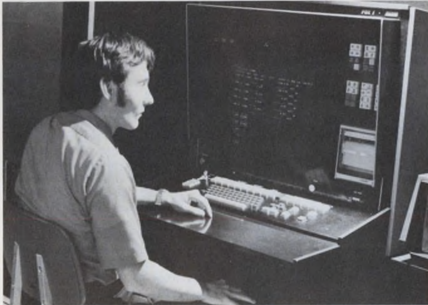
Control panels for process control systems (top) sometimes extend 200 feet. Replacing these panels now are CRT displays such as Foxboro's Fox 1 that present only the portions of the system that need attention.
