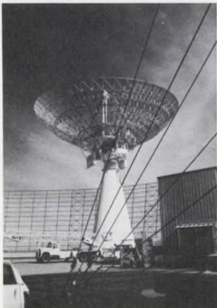
RAM vhf/uhf radar measures cross section of reentering payloads.
