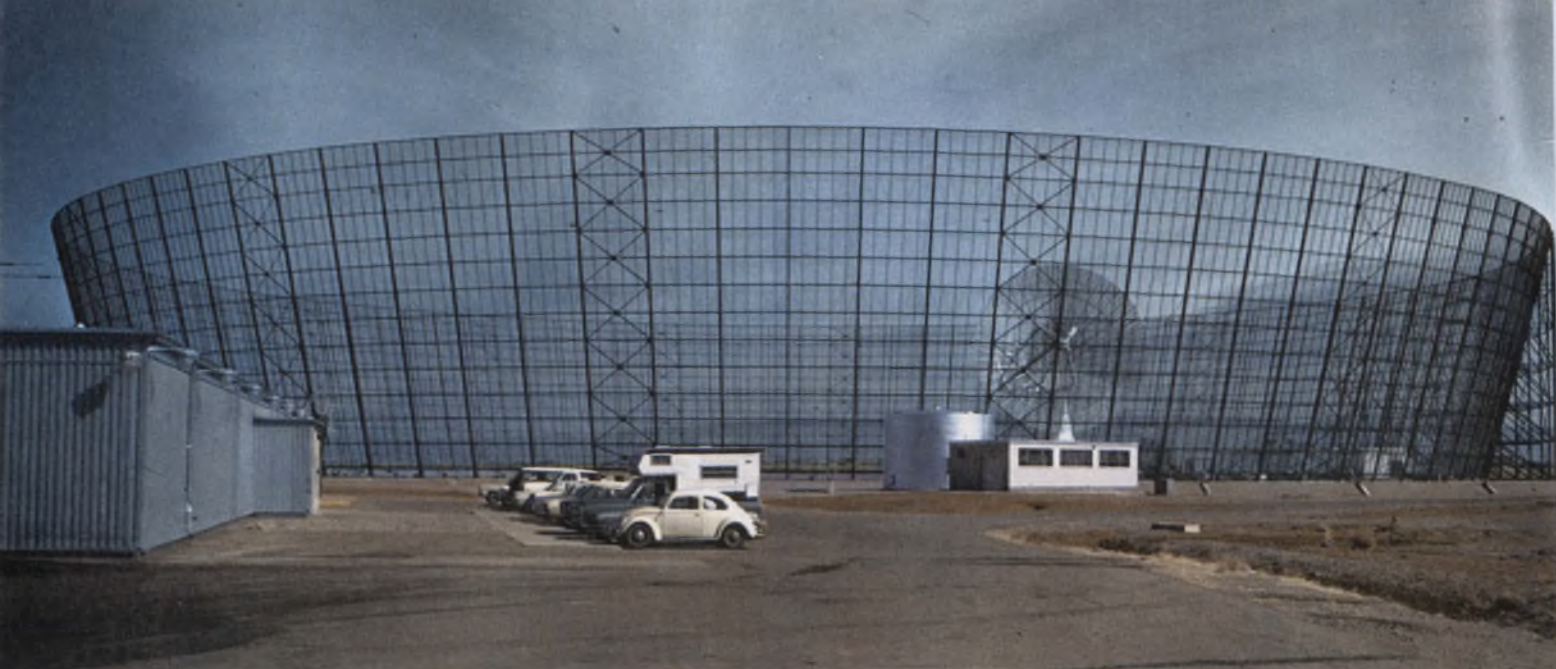
A 105-foot steel fence allows vhf radar 10 extra seconds of clutter-free data from reentering payloads.
