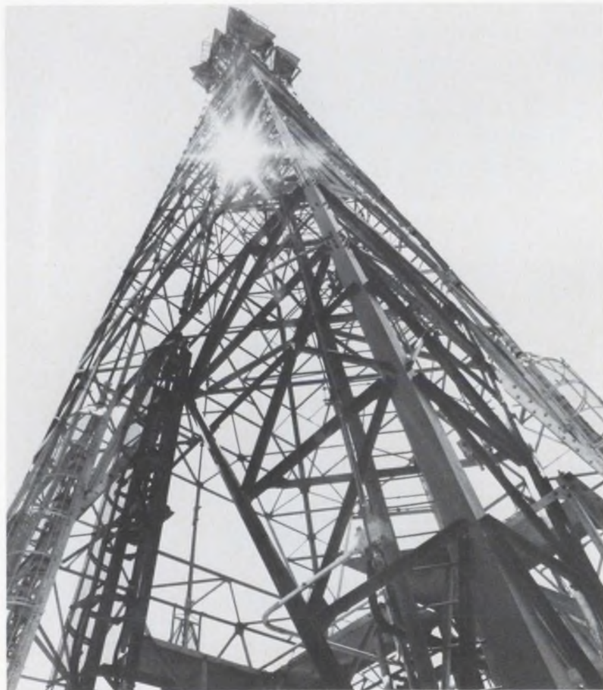
Radio relay tower for Bell's TH3 microwave system. TH3 transmits 10,800 simultaneous telephone conversations.
