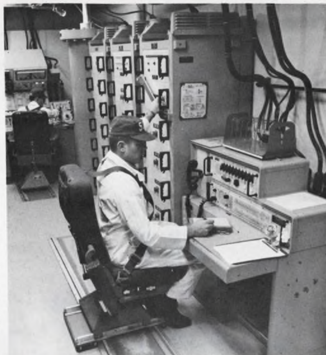
SAC missile team monitors Minuteman launch from Vandenberg AFB. On-board guidance computer continuously reports on the ICBM's status. If a fault is detected, the missile control center, some miles away, is alerted automatically.
