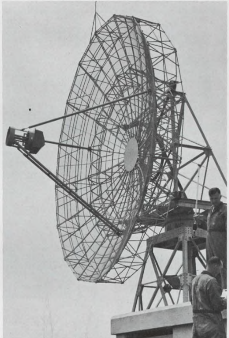
'Chirping' (pulse compression) betters radar range and resolution but keeps peak power down. Page 23
