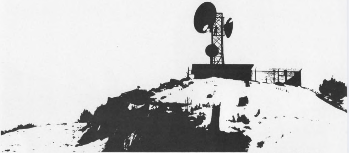
Microwave communication systems serving much of the free world.
