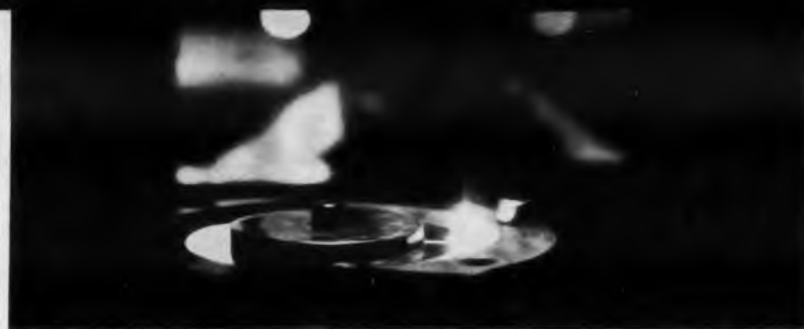
Electron-beam welding in a high vacuum was one of the recent electronic developments useful in machine design described at the 1960 Design Engineering Conference. This welder was developed by Air Reduction Co., New York.
