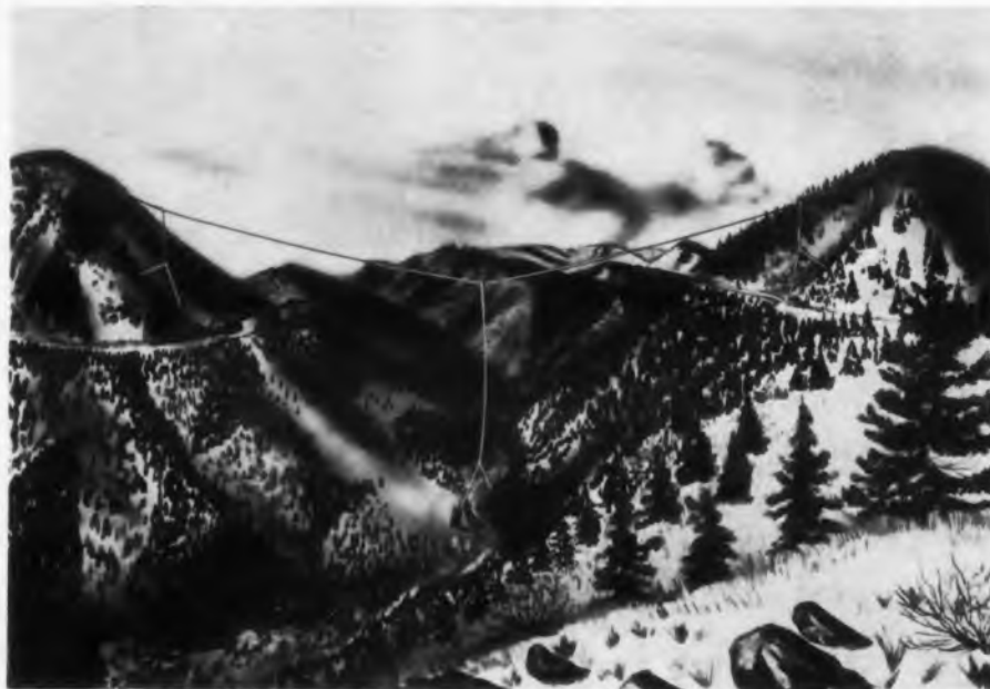
Artist's conception of the antenna across Sunset Canyon for National Bureau of Standards new-20 kc standard frequency broadcasts. The copper-coated steel cable weighs more than a ton, stretches 3,400 ft from anchor to anchor and 900 ft above canyon floor.
