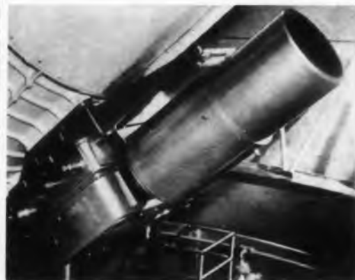
Infrared Rapid-Scan equipment for inflight spectral analysis of missile plumes is in use on the Atlantic Missile Range.
