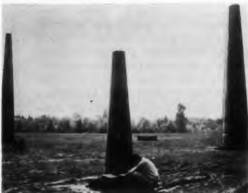
Rayon antenna tower has just been erected by technician in foreground. Developed by the American Electronic Laboratories, Inc., the tower is raised by inflation with a few pounds of air.
