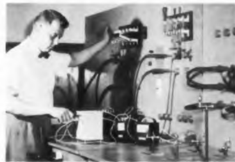
Preliminary testing of foil-wound transformer.
