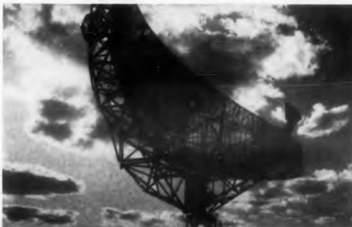
WAYLAND LABORATORY engineers developed this 40-foot L-band antenna to extend the range of radar.
