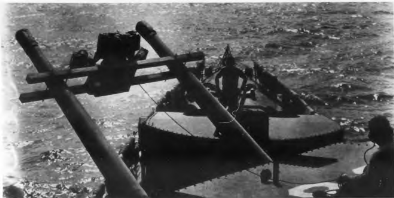
Spectral Meteor Camera was one of the major instruments used in "Operation Gaslight." It is made up of a cluster of six-F-8 Aerial Cameras equipped with spectral gratings and arranged so as to afford a panoramic view of a large portion of the sky. This meteor camera is shown mounted on the 5 in. guns of the USS Stickell.
