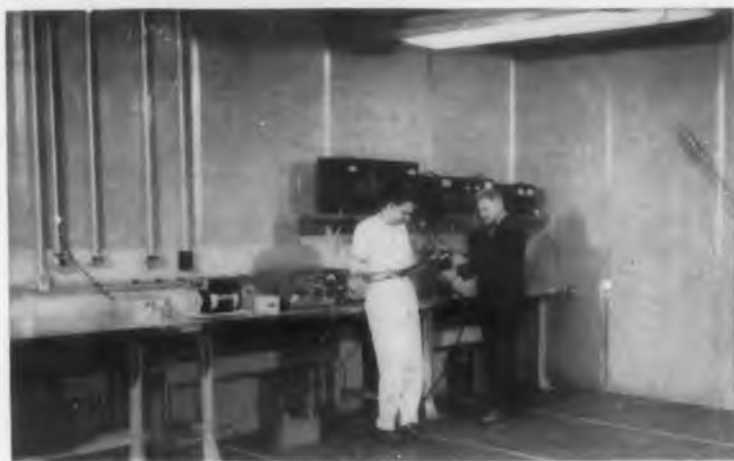
Shielded room designed and manufactured by Shielding, Inc., Riverside, N. J.
