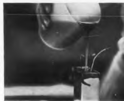
Potting transformer with Epon resin at PCA Electronics, Inc., Santa Monica, Calif.
