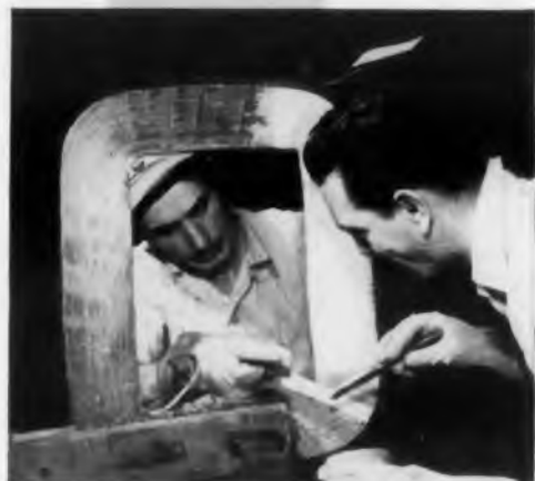
Applying Epon resin sealing compound, formulated by Epoxylite Corporation, El Monte, California, to a 400-kva transformer winding at Larsen-Hogue Electric Co., Los Angeles, Calif.
