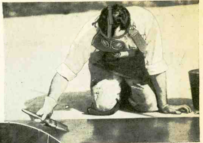
Finishing off a tennis court by means of a patent preparation which gives off a deadly gas. The workman is protected by a mask and glove. Left—When the operator of this punch press depresses the foot lever which releases the stamp, the cable attached to her wrist draws her hand back, thus preventing its accidental mutilation.
