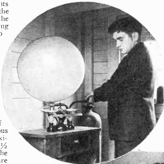
Inflating a pilot balloon preparatory to making upper air investigations. These balloons are used to ascertain wind direction and velocity at the different altitudes.
