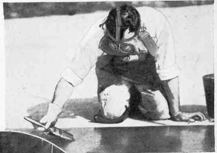
Finishing off a tennis court by means of a patent preparation which gives off a deadly gas. The workman is protected by a mask and glove. Left—When the operator of this punch press depresses the foot lever which releases the stamp, the cable attached to her wrist draws her hand back, thus preventing its accidental mutilation.
