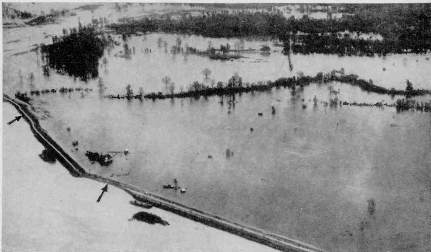
A typical Mississippi flood scene. The arrows point to weak spots in the levee.
