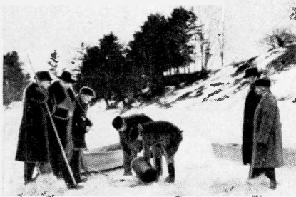
Lowering thermitite into shallow holes dug in the ice. Dr. Barnes can be seen on the left.
