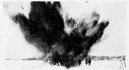
12 pounds of solite, the new ice-destroying material, reaching under the ice.
