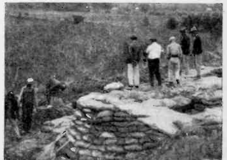
Method of treating sand boils.
