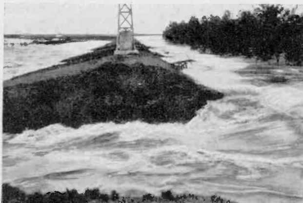
Flood waters bailing through a break in the levee.
