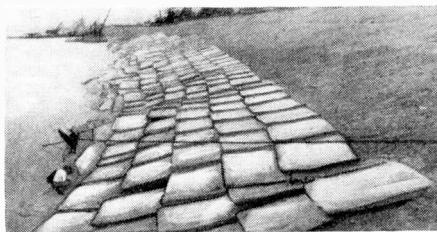
Concrete revetment. The slabs were placed on the bank by a derrick boat.
