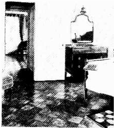
Courtesy E. L. Bruce Company This oak block floor has been chemically treated to prevent swelling, shrinkage or warping.
