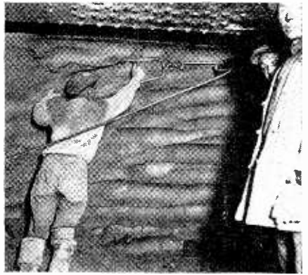
The sandhogs cut away the earth in front of the shield with small powered knives.
