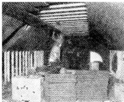
Corkboard lining will keep this attic cool in summer and easy to warm in winter. (Armstrong Cork Company.)
