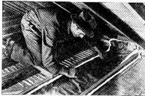
An insulating quilt of balsam wool is easily installed. (Wood Conversion Company.)
