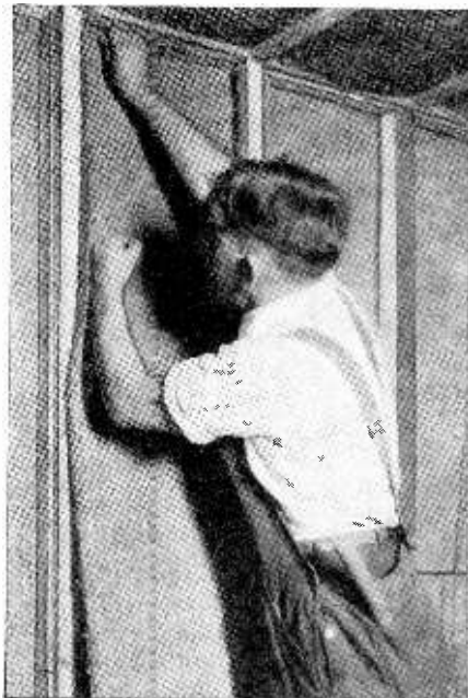
Flexible insulation between studs adds to home comfort. (Flax-Li-Num Company.)
