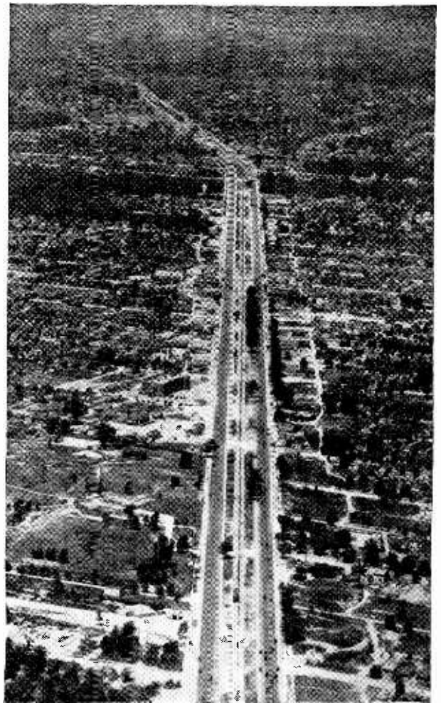
Woodward Avenue Superhighway connects Detroit with Pontiac, more than 25 miles away.
