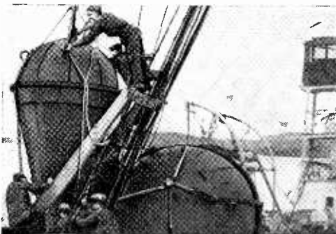
To guide the repair ship, a buoy is lowered with the end of the broken cable attached.
