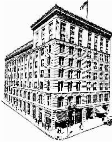
VICTOR BUILDING Our New Building Nearly Opposite U. S. Patent Office Specially Erected by Us for Our Own Use
