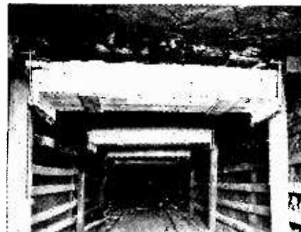
The photograph at the left shows a rock dust barrier ready to smooth a coal dust explosion. Below is a view of the rock dust shelf after the air wave has passed. The tendency of coal dust to explode is nullified by the rock dust.
