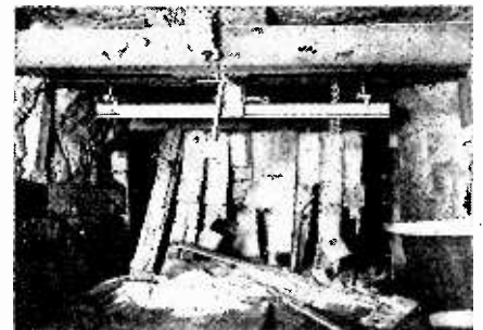
The photograph at the left shows a rock dust barrier ready to smooth a coal dust explosion. Below is a view of the rock dust shelf after the air wave has passed. The tendency of coal dust to explode is nullified by the rock dust.
