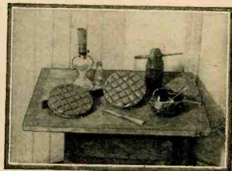
Above—The tools and apparatus used for grinding and polishing the glass.
