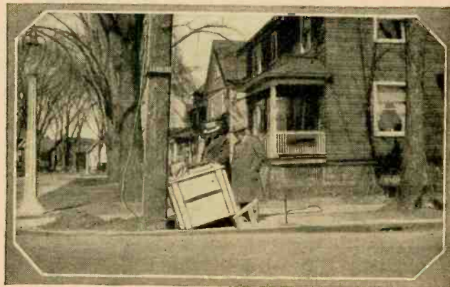
The utilization of X-rays for detecting defects in standing trees has been made possible by apparatus perfected by the Eastman-Kodak Company. Wire bearing poles have also been studied with the new outfit and imperfections within the pole or tree revealed. The above photo shows a pole being X-rayed.—N. C. McLoud.
