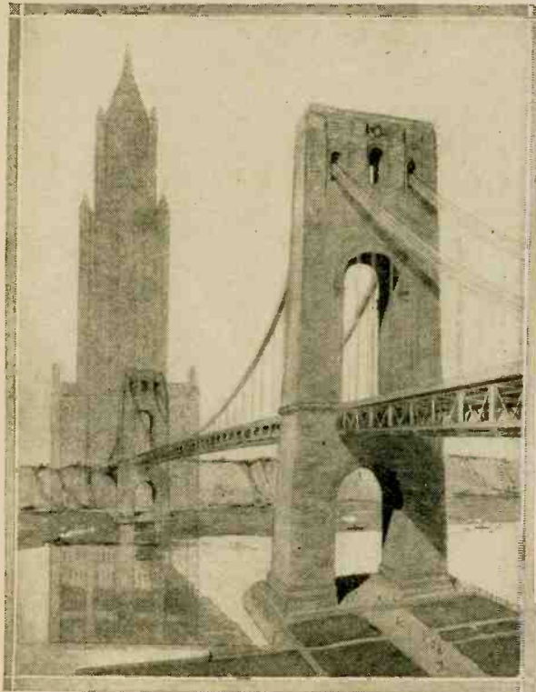
The main elements of the bridge will be the great span across the river, the supporting towers and approaches. Above one of the towers is compared to the Woolworth Building which is 792 ft. 1 in. high. The bridge towers will be 650 ft. in height.
