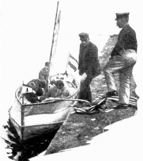
A new German invention, a collapsible rubber life-boat, is shown above. The boat will hold twenty persons, and is propelled by a four horsepower motor, as well as being fitted with a mast, sails and oars. It may be inflated by a pump or bellows. Herman Meyer, the inventor, is shown operating the bellows.
