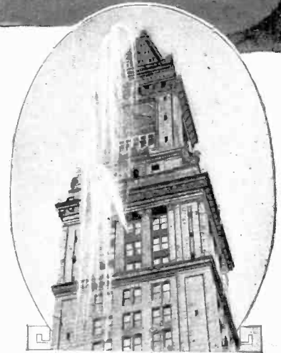
A high pressure test was carried out on the Custom House tower in Boston by the fire department. The hose projected a stream of water 500 feet above the street level under a pressure of 280 pounds.
