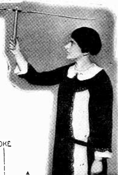
Above Miss Adele Frank is shown with the small antenna which is used in exploring the radio field for power. Note the size of the antenna and the position of the flashlight bulb. The simple apparatus used for the transmission of the radio power is shown at the left. A tube with an output of 35 watts was used. Note the size and novel construction of the short-wave transmitting aerial.
