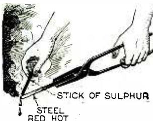
Touch a stick of sulphur to a red hot piece of steel and it will melt as easily as lead. Iron if heated white hot will act the same way. — Vernon Miller.
