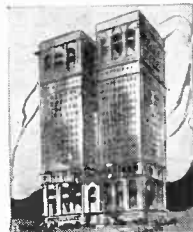
Never before has the world seen anything like the building boom of today. And this has created an enormous demand for real Draftsmen, capable of designing and calculating original work. I will prepare you for one of these fine positions at home, in your spare time.
