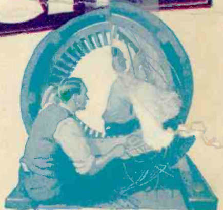
Student Winding Stator in COYNE Shops
