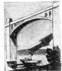
The demand for Draftsmen experienced in Structural Steel and Concrete work is enormous. All large structures require Draftsmen who can calculate and design the steel and concrete framework. Many positions open, enormous salaries offered.
