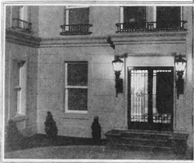
The beautifully designed and well lighted entrance to this model apartment house is shown in the photograph directly above. The lighting equipment, although operated from a six-volt source of power, was so designed that perfect results were obtained. The specially built fixtures lost none of their effectiveness through being operated at this low power. As can be seen in the photograph at the right, even tiny street lamps were included in this exhibition.
