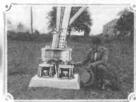
structional methods used for these tall masts can be gained from the photograph. They rest upon solid concrete bases sunk many feet in the earth, but interposed between the actual steel of the mast and the concrete are huge porcelain insulators as shown in photograph in the lower right-hand corner.
