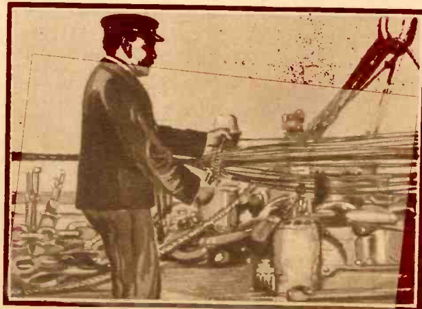
Above: Splicing a section of the trans-Atlantic cable. The workman is putting on the steel armor layer.
