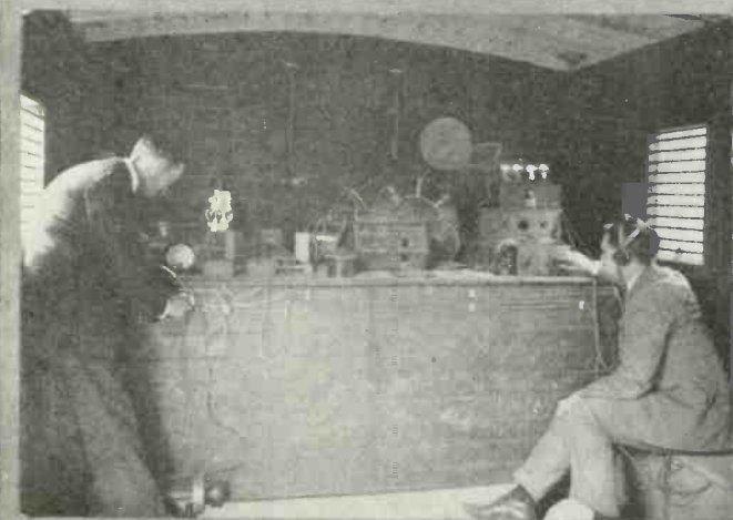
Here are shown engineers representing the Compagnie Telegraphique making experiments at the "fixed" station shown in the photo at the top of the page. Power for operating the transmitting set was obtained from a small motor-generator working on a storage battery. A number of different circuits were used and the results obtained with each were carefully tabulated.
