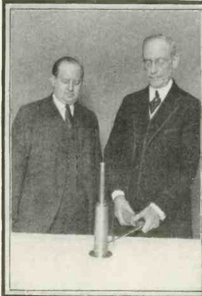
New Liquid Air Jack Shown at Left Will Lift 30,000 Pounds. It Was Invented by Walter S. Josephson of New York Who is Demonstrating it.
