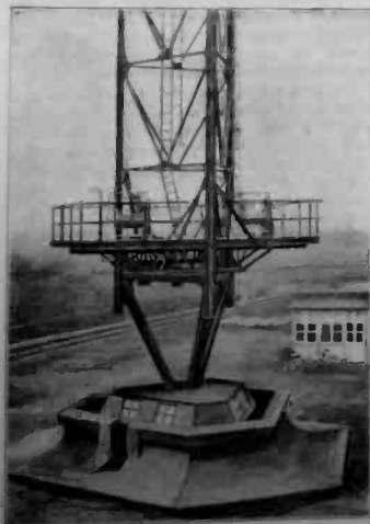
Strange as it may seem, the gigantic 700 foot Radio Towers Employed at the Station in Nauern, Germany, are Balanced on Their Points. The Towers Themselves are Triangular in Shape and Each One Weighs 792,000 Lbs., and Rests on a Foundation of Porcelain. The Complete Installation is Shown Above.
