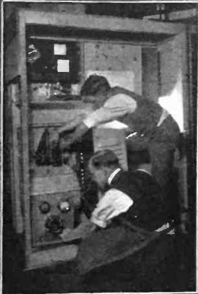
Testing Electrical Alarms and Other Protective Devices in a Safe.
