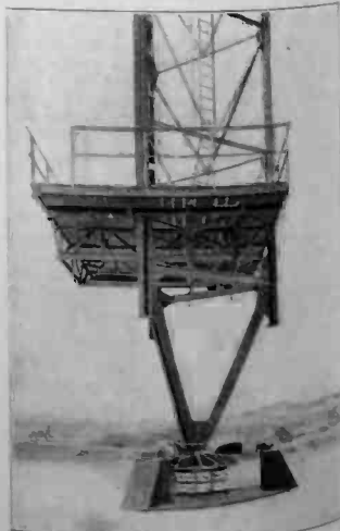
A View of the Tower Base is Shown Above, with the Outside Casting Removed. The Extreme Point of the Tower is movable Upon its Foundation, so that it can Sway Slightly When Affected by High Winds. This is Necessary to Eliminate the Possibility of Breakage in a High Wind. A Complete Description of This Base is Given in the Text.
