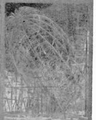
The Schutte-Lanz airship in the course of construction in German factory, less the external skin.
