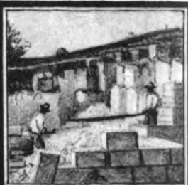
Mining Animal Rock (Coral Rock) that Forms Nearly all of the Island of Bermuda. Some Rock Can be Easily Worked Without Using High Explosives, But Other Rocks, Again, Such as Granite, Are Extremely Hard to Quarry.
