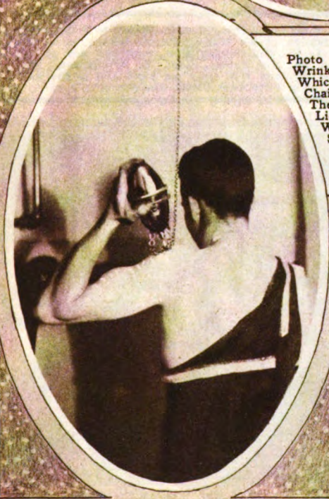
Another Useful Science Wrinkle Applicable to Home Needs. This Consists in Placing an Electric Light Bulb in the Oven Which Provides Just the Right Amount of Heat for Bread Raising. A 60-Watt Bulb Will Usually Provide the Proper Amount of Heat, But This Will Depend Somewhat Upon the Size of the Oven.
