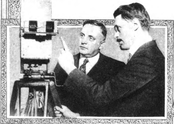
The Photo Above Shows the Inventor (at Right) and His New Binocular Vision "Movie" Camera Which Is Said to Solve One of the Most Absorbing and Difficult Problems in Motion Picture Work—That of Providing a Picture Having True Depth and Perspective. The Inventor Is P. John Berggren of Swedish Extraction, But Now of Chicago. This Machine Would Seem Then to Give the Effect We Have Long Sought—Real Stereoscopic Motion Pictures in Which the Images Stand Out in Relief.
