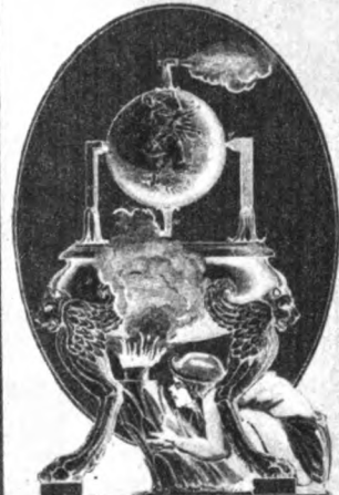
HERO'S ENGINE WITH BOILER
