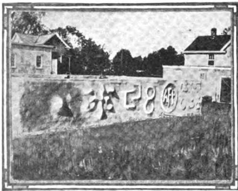
Illustrating Vividly What May be Accomplish in Building Out in Relief, With But One Application of the "Cement Gun."
