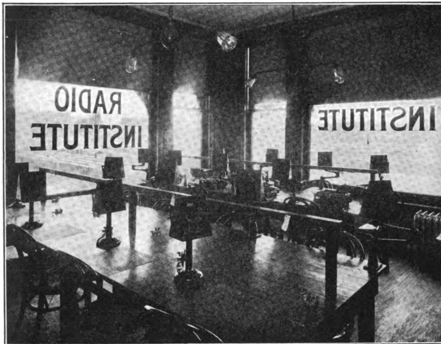
If You Would Become an All-around Radio Operator Capable of Holding Down a Land Station Berth, It Is Necessary to Learn Land-line or Morse Code Telegraphy as Well as the Continental Code Employed in Radio Work. This Illustration Shows a Section of a Radio Institute Devoted to the Study of Sounder-work. Each Sounder Is Enclosed in a "Resonator" Which Will Lie Close to the Student's Ear Not to Confuse Him by Hearing the Sounds from Other Nearby Instruments. The Student Is Taught to Copy the Message Directly Upon the Typewriter.
