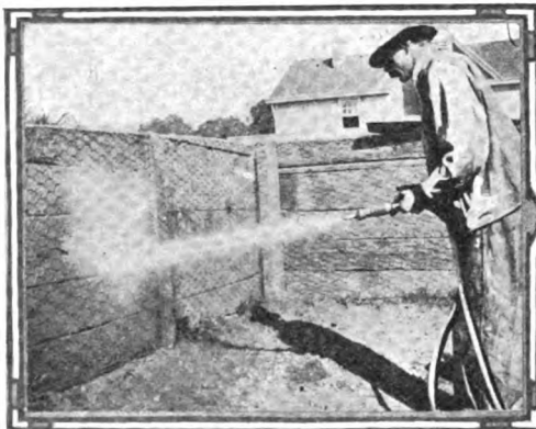
Illustrating Vividly What May be Accomplish in Building Out in Relief, With But One Application of the "Cement Gun."
