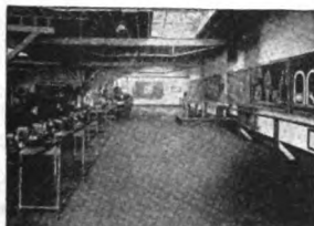
Showing part of electrical dept.
