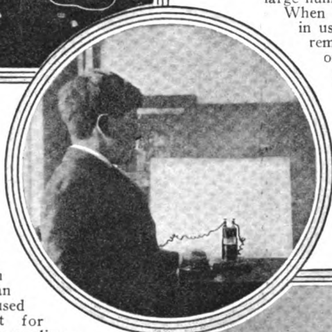
Electrolysis of Sodium Sulfate Solution, Using the Bichromate Cell as a Source of Current.
